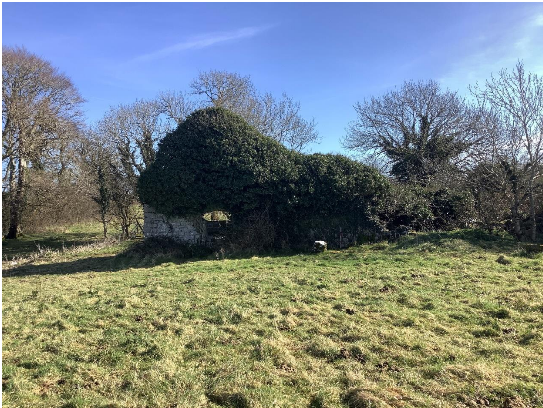
Plate 11-7: View from southern ELAR boundary looking east towards northernmost outbuilding located towards centre of site.
