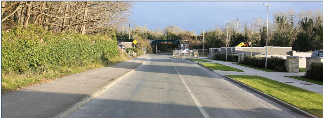
Plate 12-12 View to the south-east along the Rosshill Road, Galway-Dublin trainline crosses the bridge in the centre of the image and the (under construction) Ross Alta development is seen to the right of the road.
