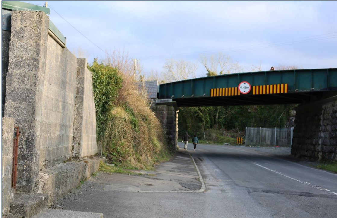
Plate 12-23 View to the south from the L5037 Rosshill Road showing the train bridge approximately 35 metres north of the site.
