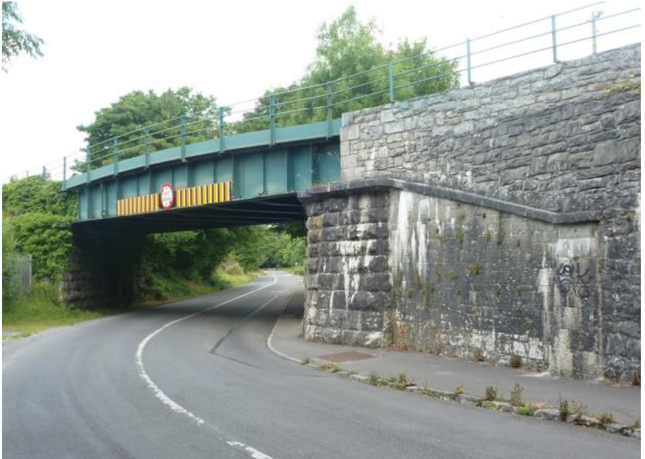
Plate 11-17: Protected structure 8806, 19 th century railway bridge. Photo courtesy of Galway RPS.
