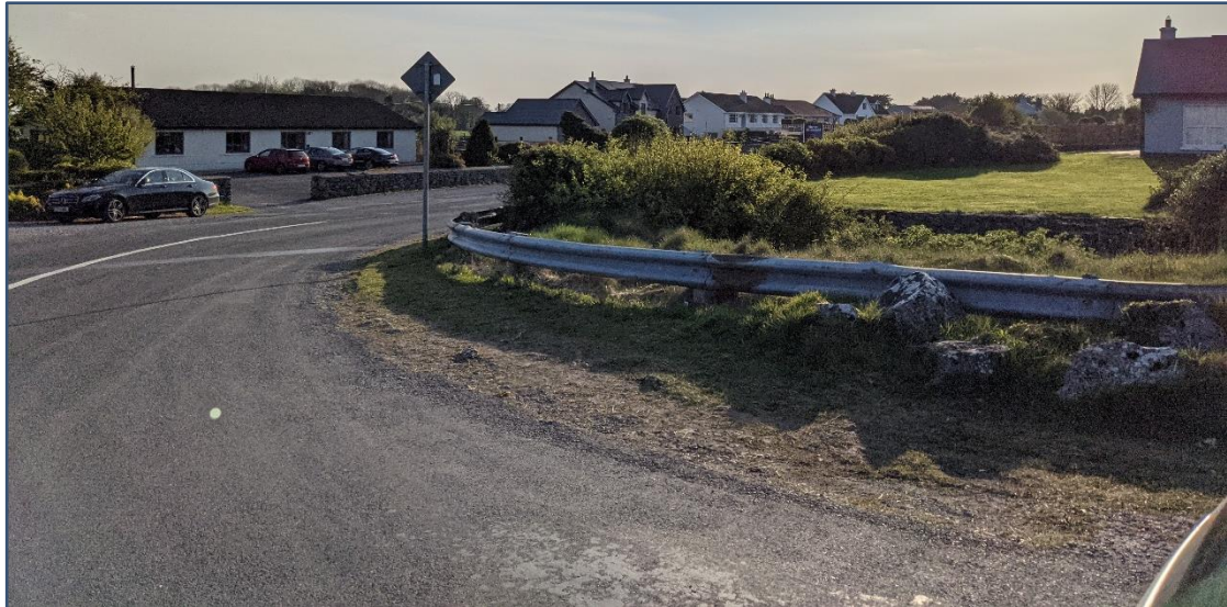
Plate 12-18 View west towards the Proposed Development at the junction between the Coast Road and Rosshill Road at the western extent of the GCDP Protected View V8.
