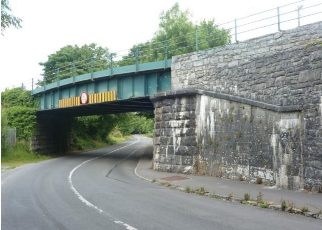
Plate 11-1: Protected structure 8806, 19 th century railway bridge to the north of the proposed development site along public road.
