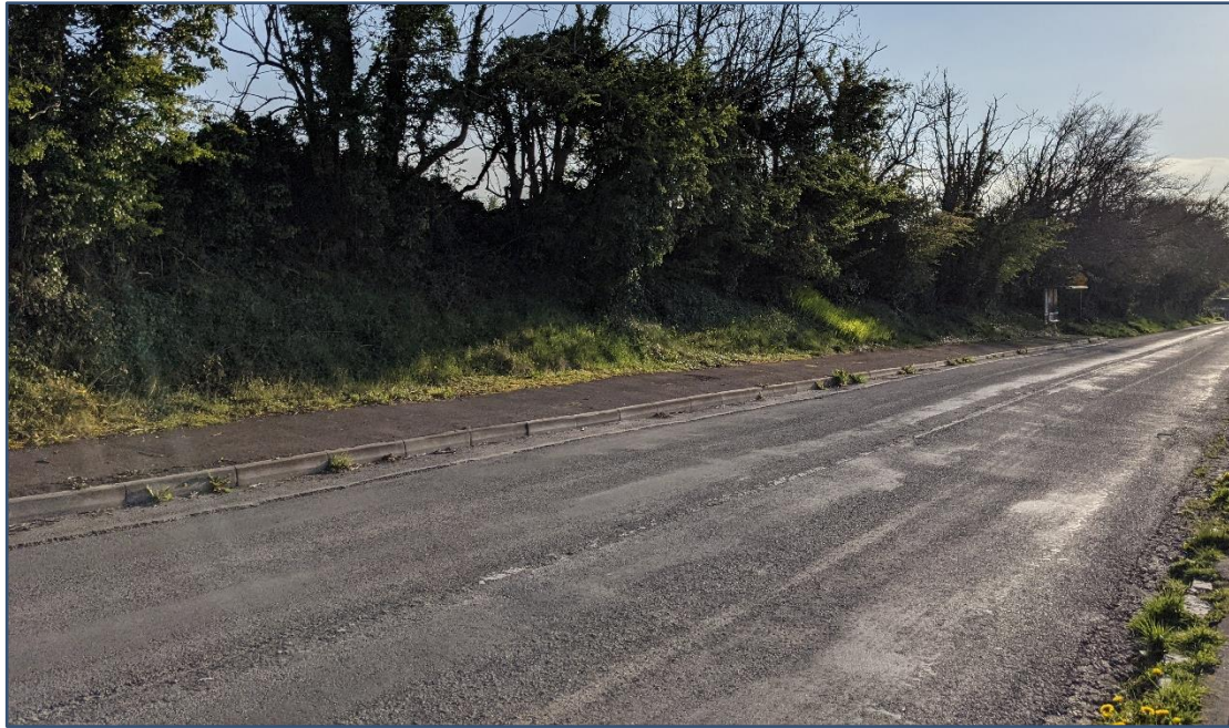
Plate 12-8 Steep embankment along the northern boundary of the site on the Rosshill Road.
